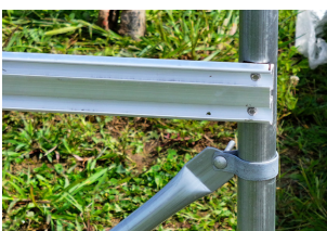
Double wirelock at end bow.
