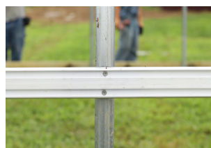
Double wirelock at bow
